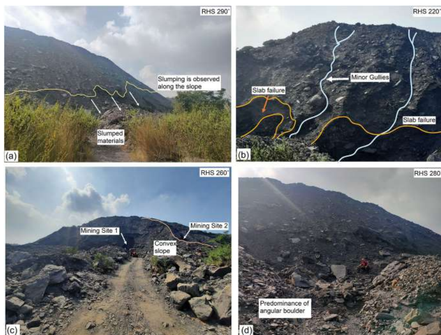
Fig. 2 Dump site at location 1. a. Slumping along the slope. Slumped material deposited at the base. b. Slab failure at the toe of the slope. Minor gullies developed along the slope. c. Overall geometry of the slope is convex. Two mining sites noted. d. Predominance of angular- boulders at the dump site
