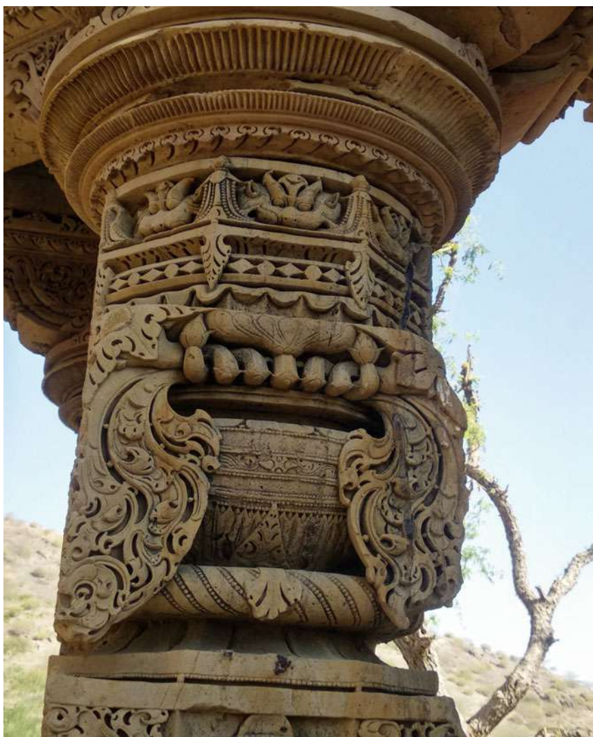
Rep. Fig. 7 Detail Decorations (Floral motif) at the partially damaged pillars of the Mahamandap of the Vishnu temple (Temple no. 6)
