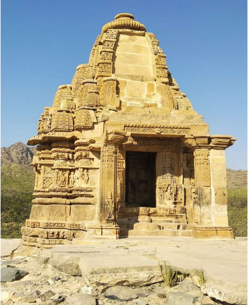
Rep. Fig. 5 Frontal image of the partially damaged Shiva temple (Temple no. 5)
