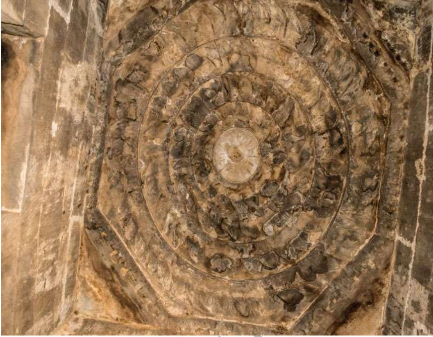
Fig. 18 Leaching of water in sandstone at the ceiling of the Shiva temple (Temple no. 1)
