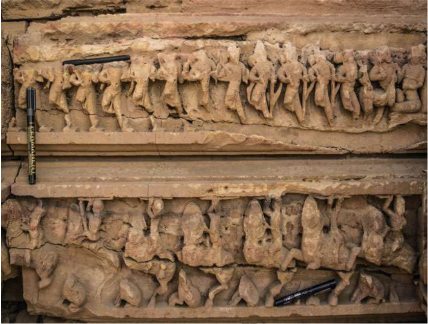
Fig. 24 Weathering of the Someshwar temple wall (Temple no. 2) (black pen of length 14 cm)
