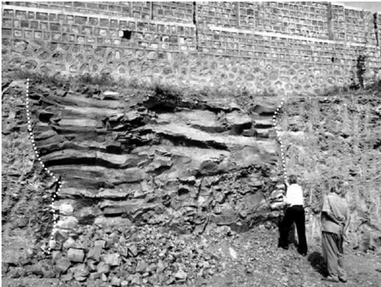
Fig. 14. Exposure of the Majnu Hill dyke ( D_4 ) showing no displacement.
